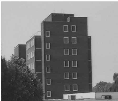
Fig-1 Image of a real building
