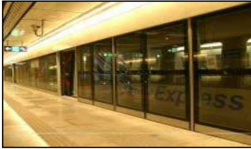
Fig. 3: Platform screened from the tracks
